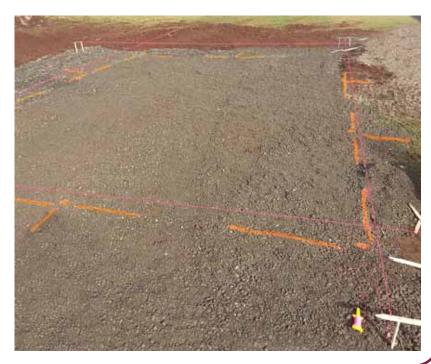
**Step Two (B):** Now just like in Step Two A, you will set the kickers up identical two have two vertical strings that align up.
