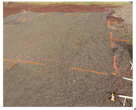
**Step Two (A):** make eight "kickers" (see A). Set two of the kickers 3' beyond one of the spray paint marks to line up one of set of marks
